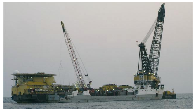
Figure 7. Construction of offshore pipeline.
