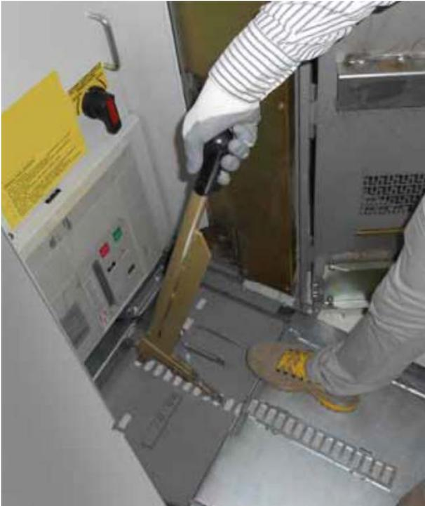
**Figure 2.** Open-door racket lever circuit breaker racking-in operation
