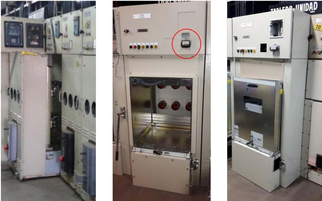
**Figure 8.** Retrofill motorization upgrade for minimum oil breaker
