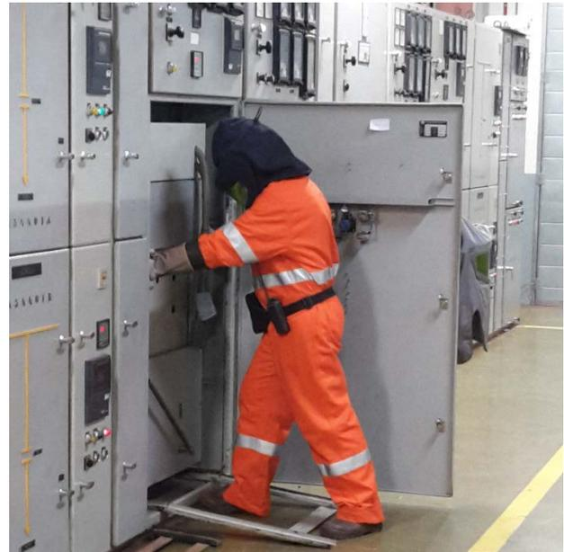
**Figure 1.** Open-door circuit breaker racking-in operation
