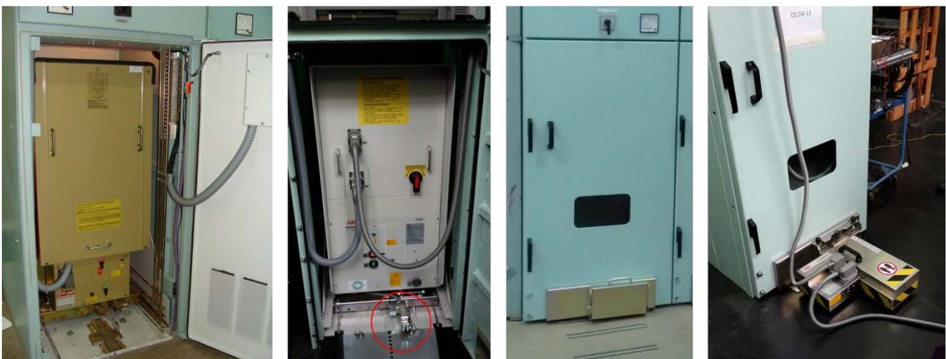
**Figure 7.** RiR motorization upgrade for a racker type air-magnetic breaker with linear operation
