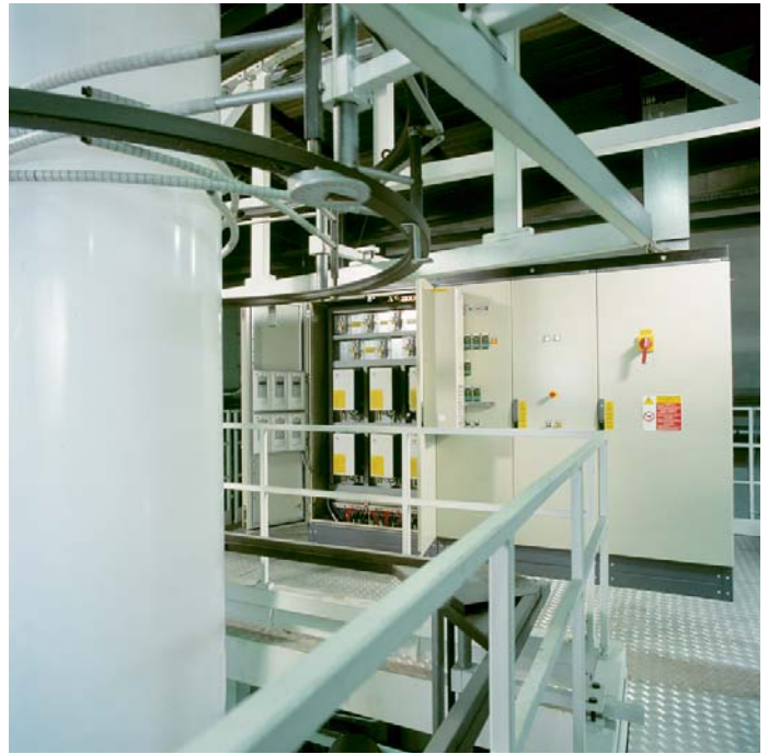
ABB industrial drives installed in the cabinets.
