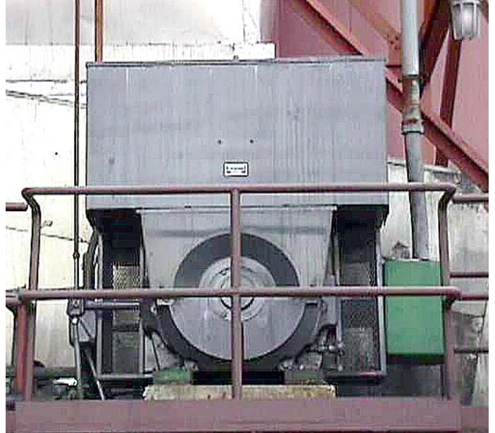
The 20 year old fixed speed fan motor, now controlled by the ACS 1000, operates more efficiently and quieter.
