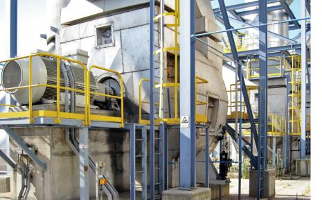
01 The three ID (induced draft) fans at Valorsul's WtE plant are now controlled by ABB's ACS2000 variable speed drives.
