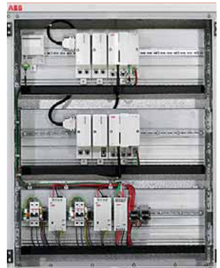
4 The AC 800M controller mounted in a rack cabinet
