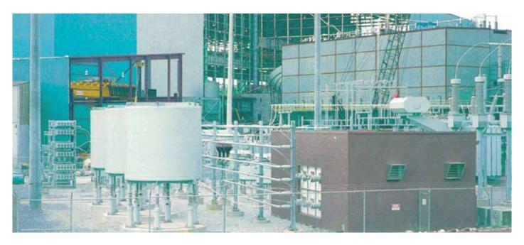
A Static Var Compensator (SVC) rated at 0–110 Mvar (capacitive) and supplied by ABB has been in operation since 1996 in Alabama Power Company's 230/34.5 kV dedicated substation located at the Nucor Steel Tuscaloosa plant in Tuscaloosa, Alabama.
