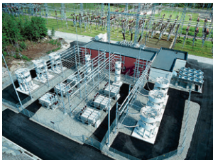
SVC works just like a shock absorber.
