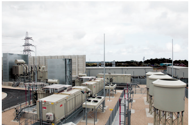
PCS 6000 (in middle) and MSR (to the right) for Westermost Rough offshore wind farm, UK.
