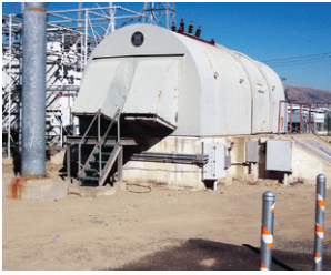
A Rotating Synchronous Condenser is a synchronous machine that is powered from the grid. It has no physical load and performs both as a generator and absorber of reactive power in the grid.
