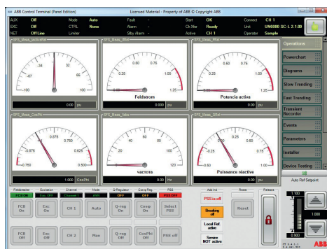
01 Excitation Control Terminal operator screen selections
