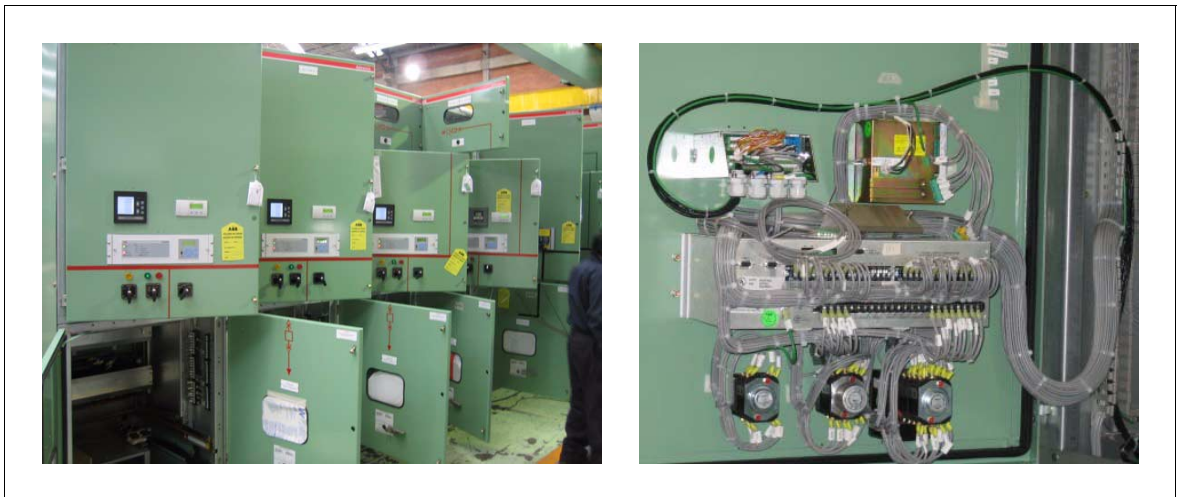
Bild 2-2: Installation the central device as panel mounting in switchgear
