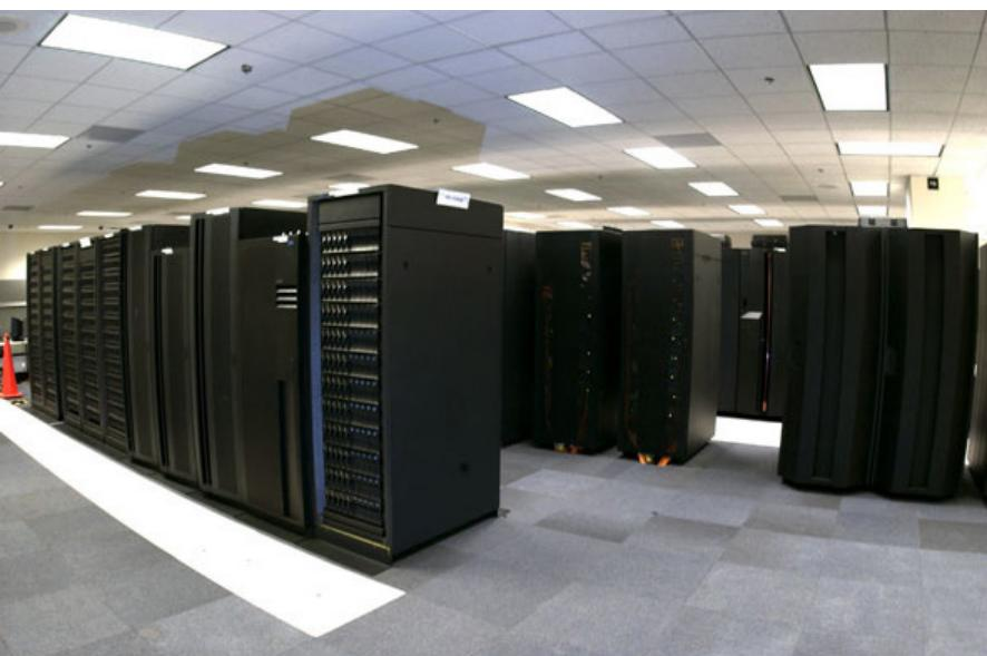
The ABB solution is installed at the National Institute of and Atmospheric Research (NIWA) in Wellington, New Zealand, where it protects the new climate modeling supercomputer and the entire NIWA site from voltage fluctuations.
