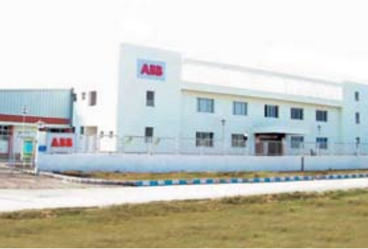
LV Distribution electricals factory, Haridwar
