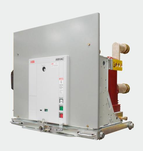
AMVAC indoor medium voltage vacuum circuit breakers with magnetic actuators are tested according to the latest IEEE standards.
