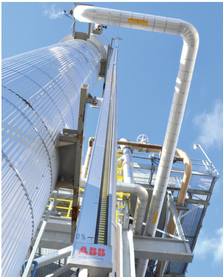
1 AO2040 emission analyzer | 2 266 pressure transmitter | 3 KM26 magnetic level gauge | 4 Multivariable transmitter
