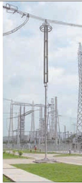
5b 500 kV DC bus arrester (2000)
