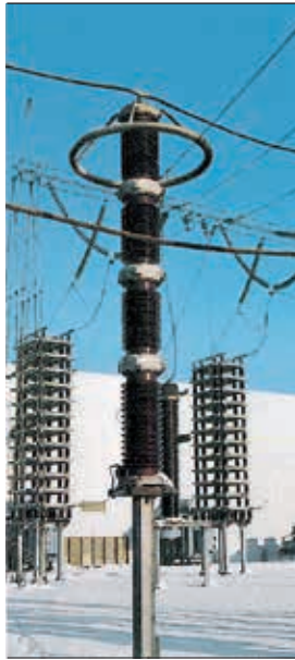
5a Gapless HVDC line arrester (1979)
