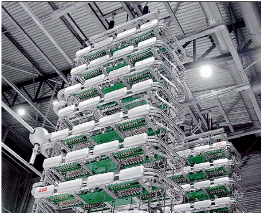
1 Valve suspended from the ceiling of the valve hall
