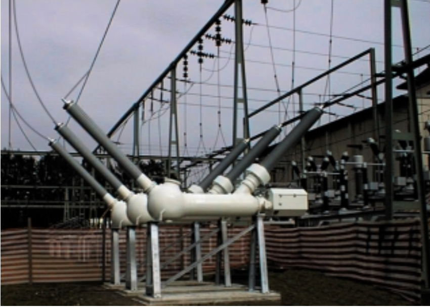
Substation extension with PASS (coupler bay)
