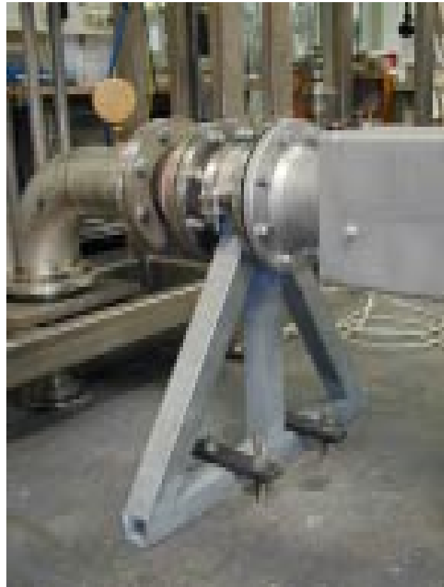
Figure 2 - Supports near inlet connection of a 6 in. Trio-Mass primary
