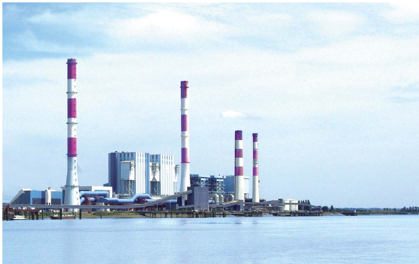
Cordemais power plant. Image courtesy of Clément Bucco-Lechat
