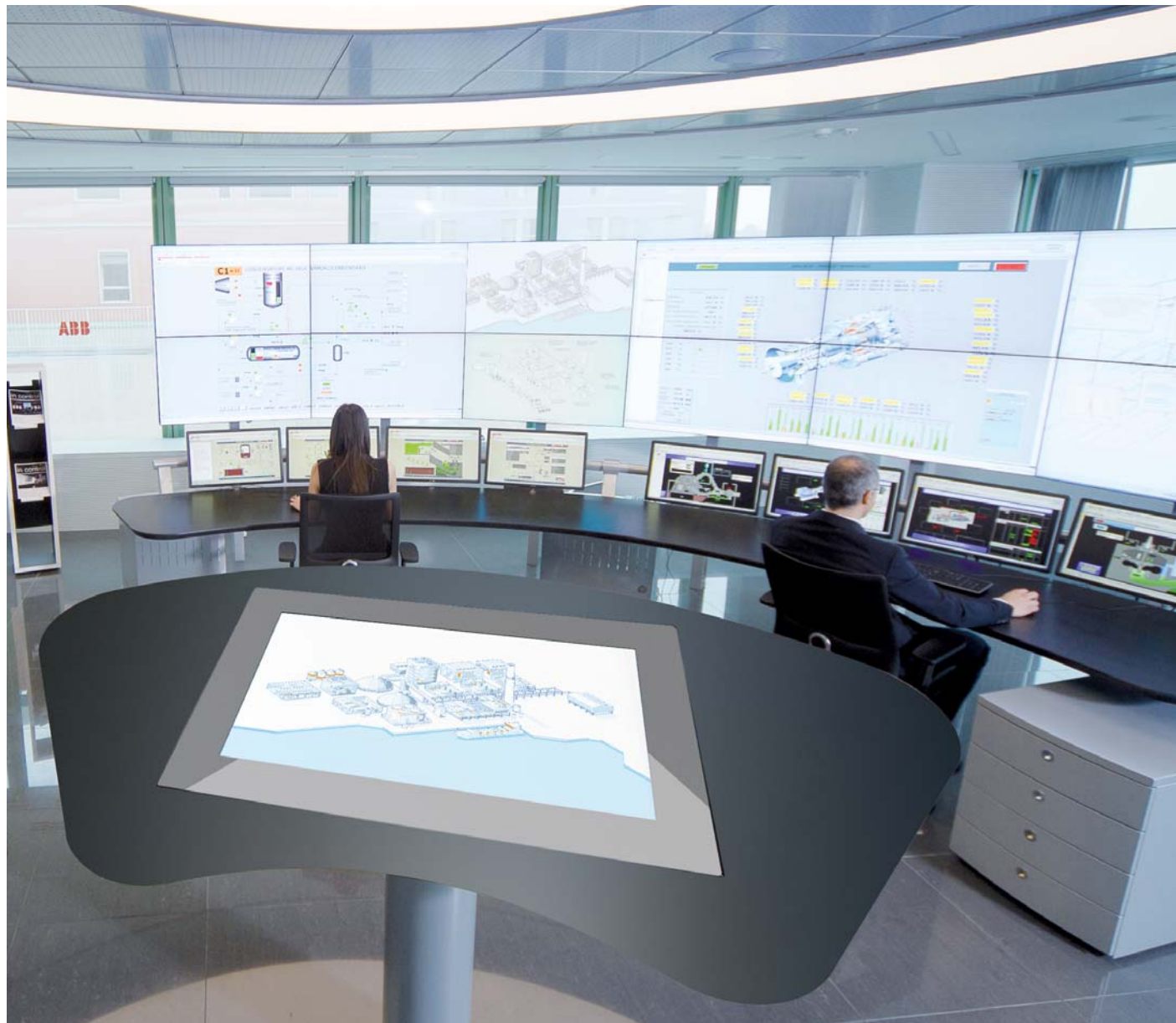
A Symphony Plus control room
