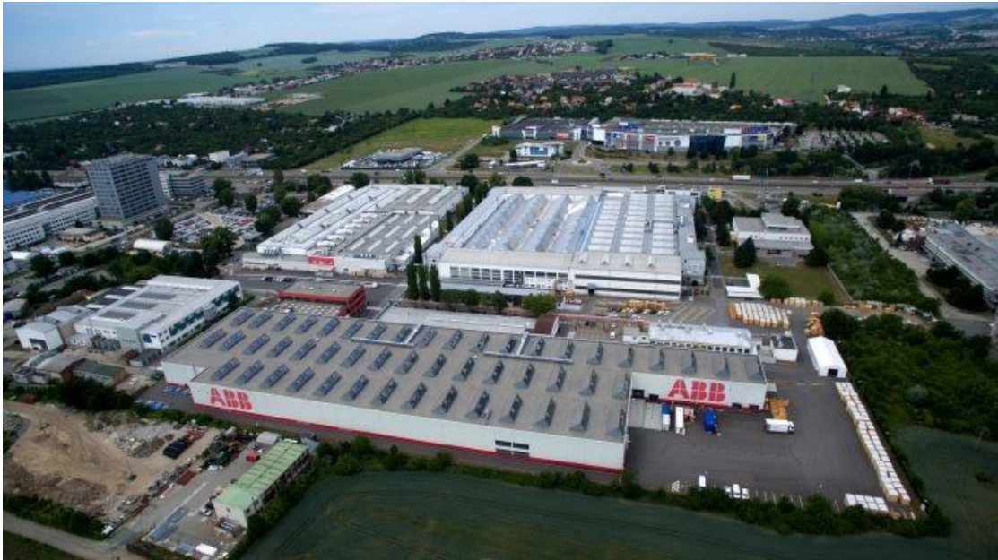
Figure 1: ABB Brno Videnska
