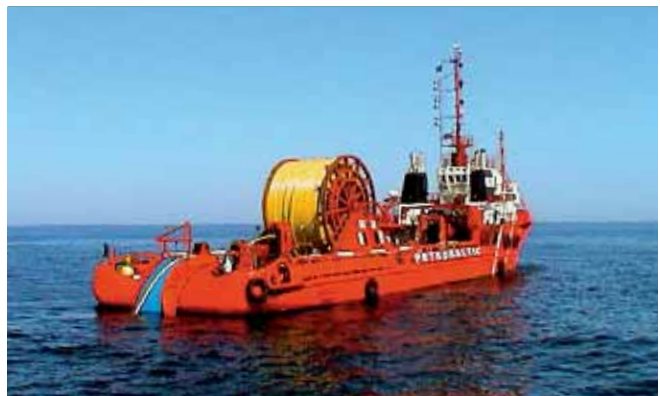
3 The gas pipeline was reeled out in 11 km sections
