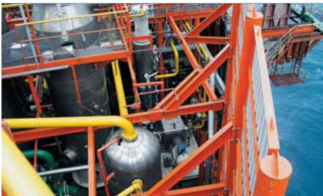
2 Initial treatment of the gas on board the “Baltic-Beta” drilling-rig – previously this gas was wastefully flared off
