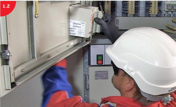
Start by removing the existing relay.
