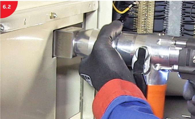
Make eight punches in two columns, side by side.
