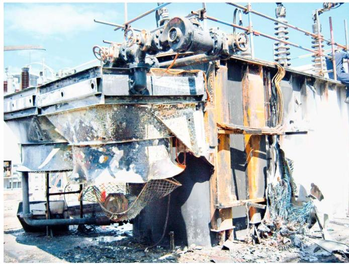
**Figure 4: A nearly catastrophic failure damaged a transformer.**
