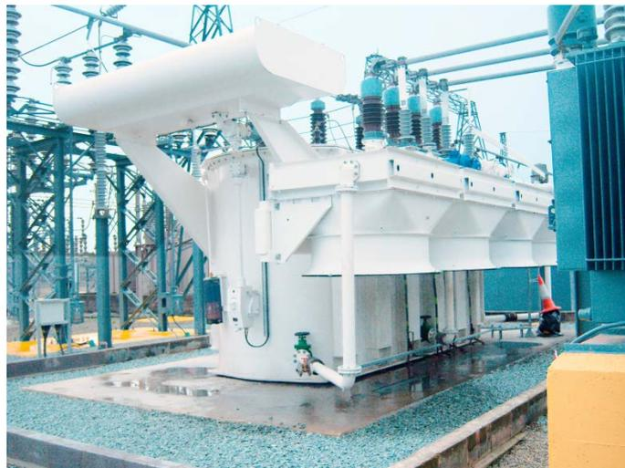
**Figure 5: The transformer (previous figure) has been remanufactured to a fully functional status.**
