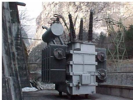
**Figure 14: 12 MVA, 20 years old generating Step-Up transformer.**
