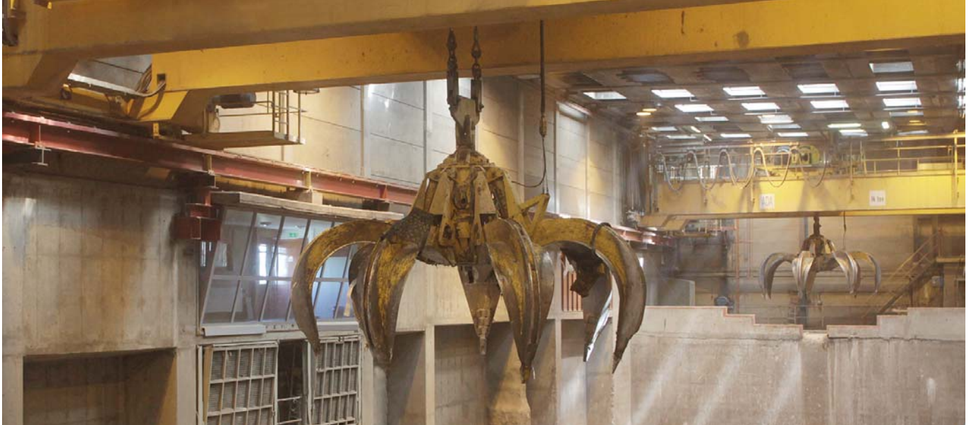
The crane's trolley and long travel movements use the ABB anti-sway control program to prevent the load swinging.
