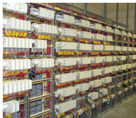
S800 I/O in electrical room (left), the central control room of the iron ore pelletizing plant (right).
