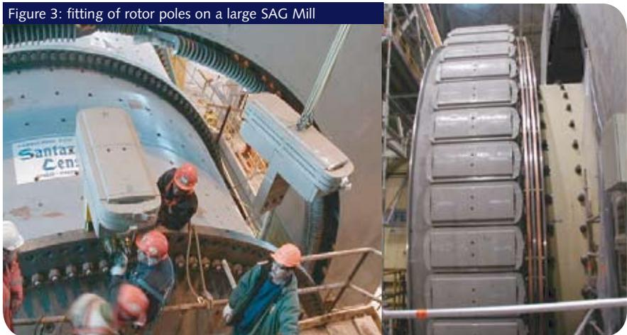
Figure 3: fitting of rotor poles on a large SAG Mill
