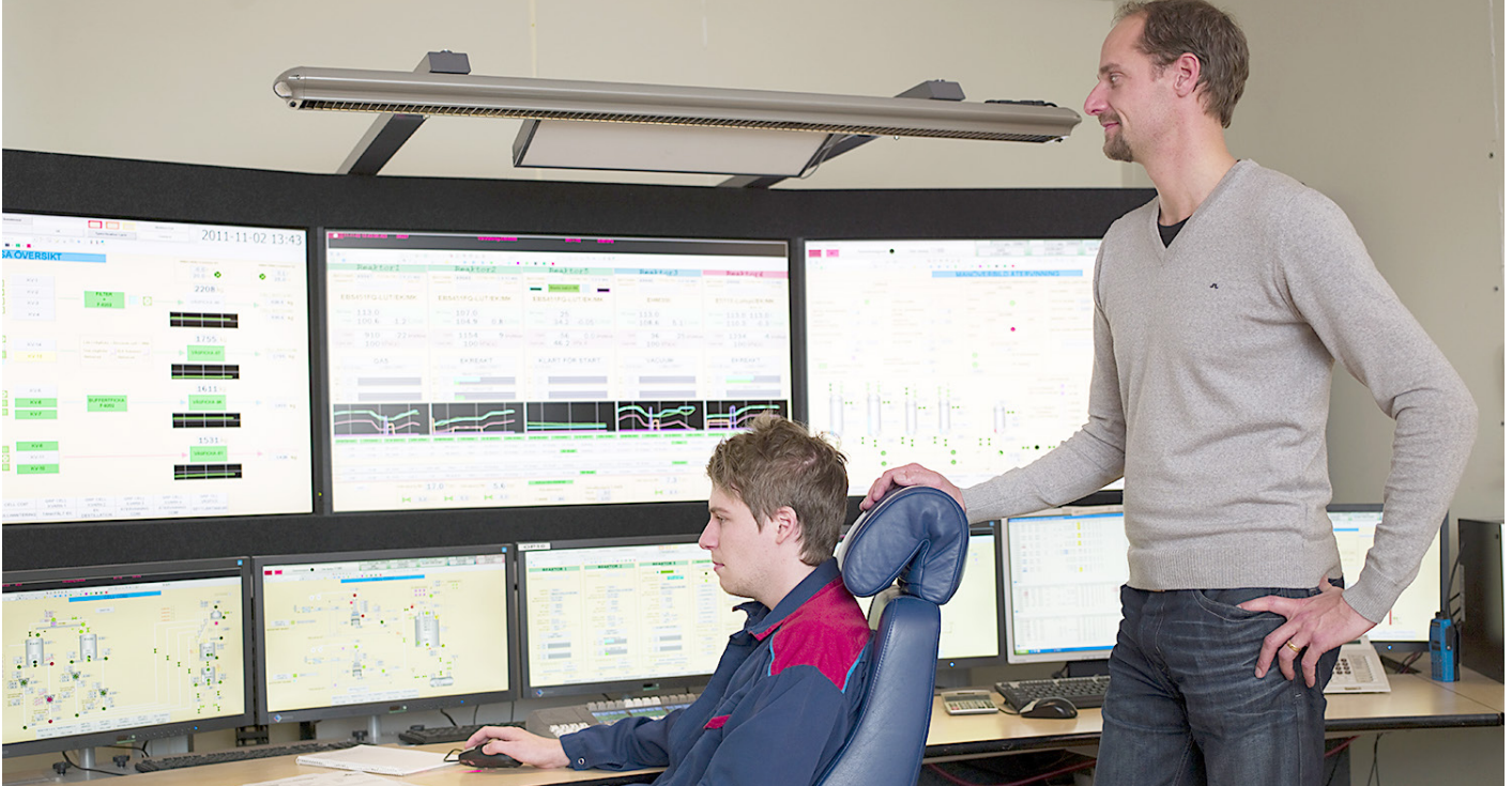
Robert Lundvall, Technical Manager at AkzoNobel Functional Chemicals in Örnköldsvik, at the Extended Operator Workplace EOW-x that has helped free up operator's time, enabling them to focus on task such as process optimization.
