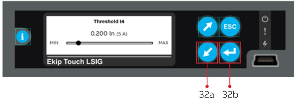
The setting range is from 0.1 to 1.0 of the breaker's nominal rating (rating plug/sensor value). Press the **Up** or **Down** buttons (32a) to change to the value in the coordination study (maintaining the press will advance the settings faster). Then press **Enter** button (32b).
