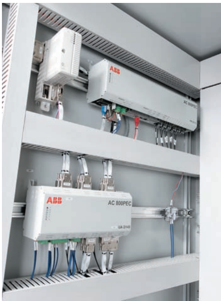
Fig. 5: AC 800PEC with the optical link connection to the Combi I/O
