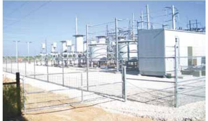
In addition, the concept of medium size SVC units distributed to critical busses in the system was chosen by AEP for the ability to apply the dynamic support close to load and the wind generators. This yields effective reactive power support during post fault system conditions and maximizes the power transfer capability out of the wind farm areas during shifting wind conditions.
