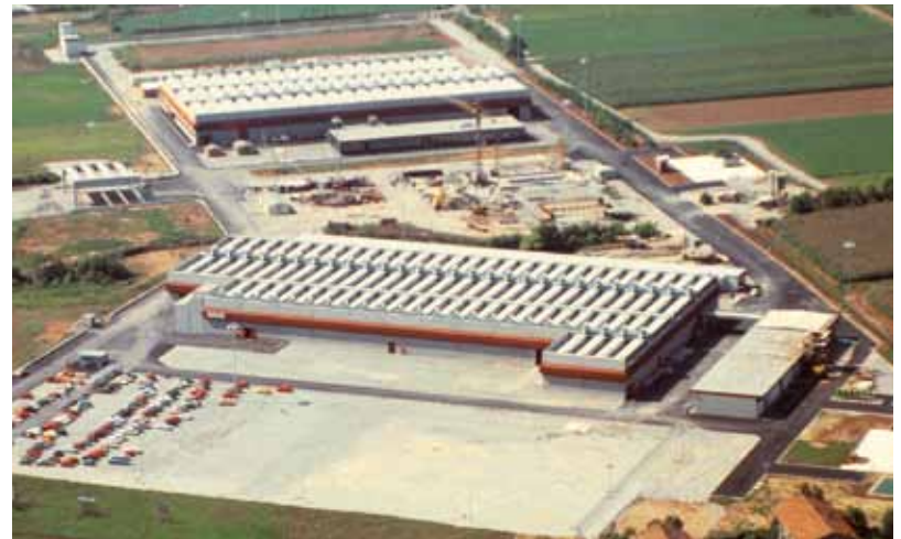
Above , the SACE SUD factory (SACE Archives, 1972); below , aerial view of the Dalmine factory (SACE Archives, 1977).
