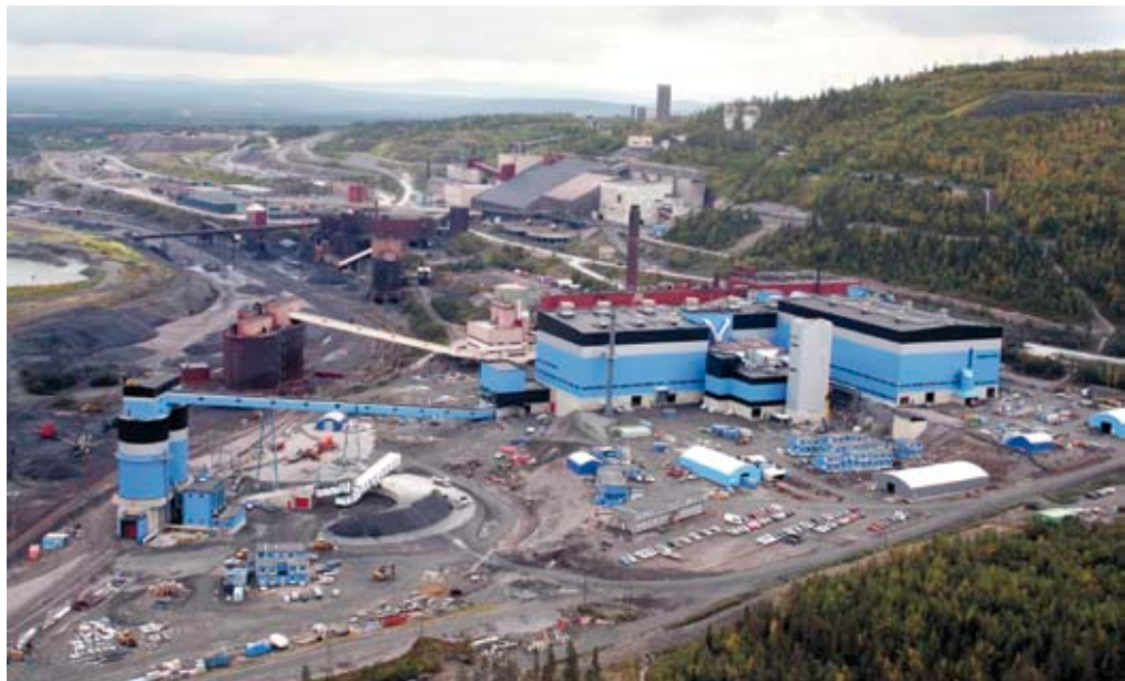
View of the new pelletizing plant MK3 in Malmberget.
