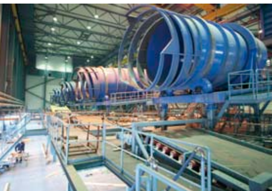
The raw pellets are formed in the balling plant of the new installation at LKAB's Malmberget.
