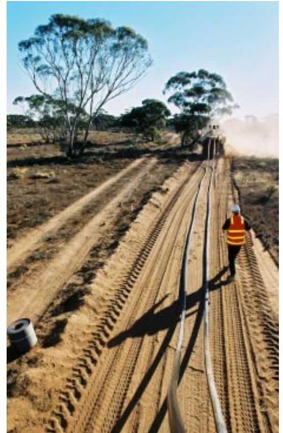
Burying of the land cable.
