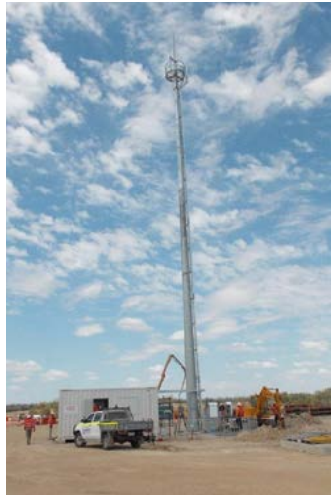
— Access point radio mast at Ruby Jo.
