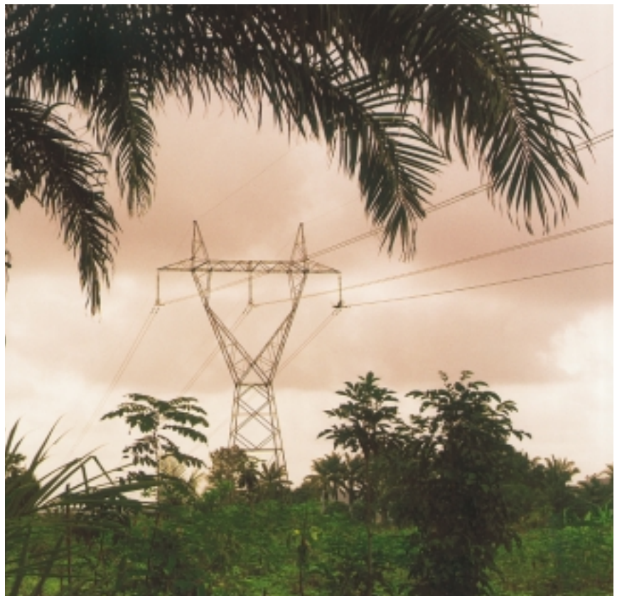
330-kV Sapele–Aladja single-circuit AC line, Nigeria (1982)
