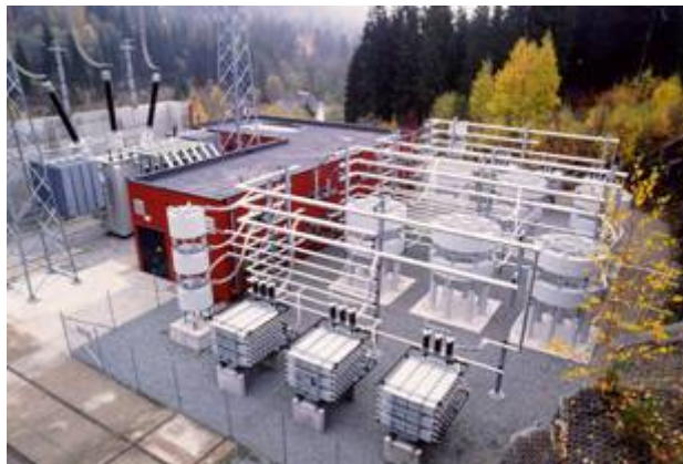
FACTS technology can reduce losses in existing lines by as much as 40%
