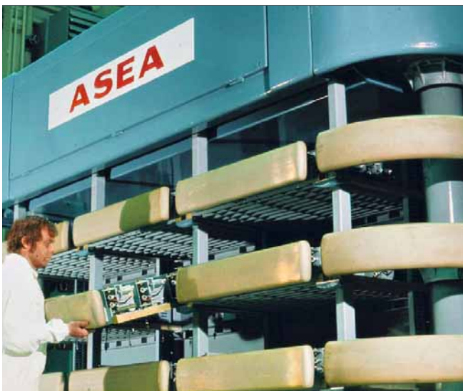
An early ASEA thyristor-based HVDC converter
