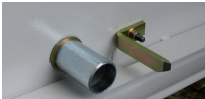
Lock installed in internal part of door
