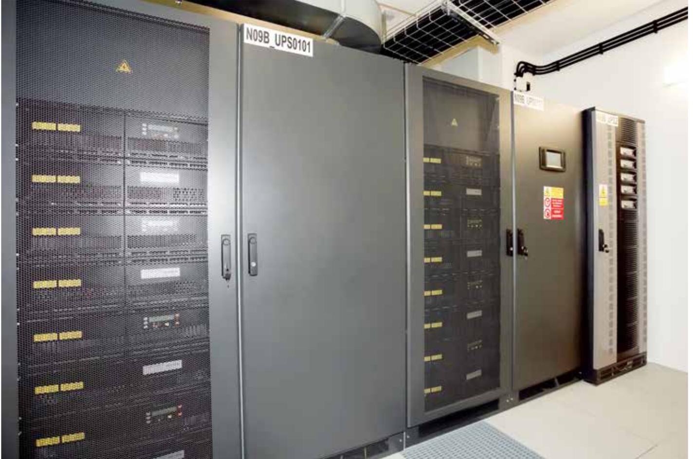
In October 2015, PRONIX finalized the development of a data center in the Czech Republic for TTC TELEPORT. With a floor area of 8,000 m<sup>2</sup>, the data center is the largest in the country. The project included a new backup power supply concept with ABB DPA UPSs.
