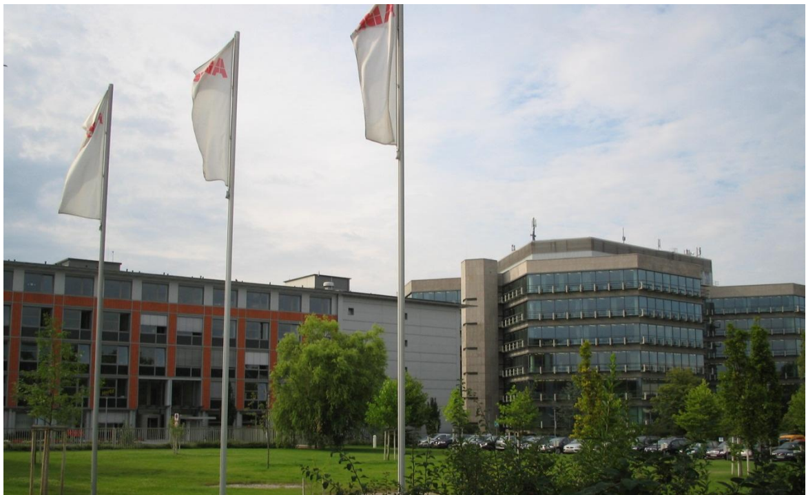
Picture 5 ABB Power Systems Mannheim training facility: red building, fourth floor
