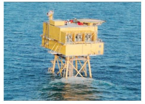
generators are automatically connected to the offshore network as they detect the presence of the correct AC voltage for a given duration. This functionality cannot be realized with classical thyristor-based HVDC transmission, as the latter would require a strong line voltage to commutate against.
