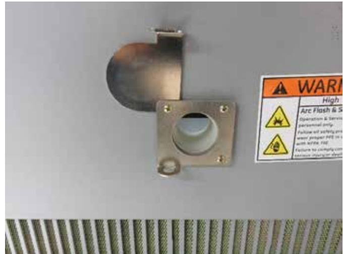
Figure 2-2: Racking Mechanism Door, Unlocked
