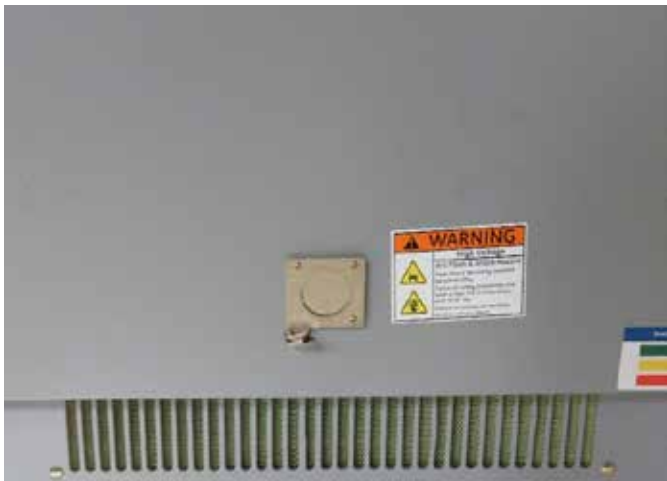
Figure 2-1: Racking Mechanism Door, Locked
