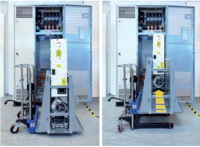
**Module lift for handling R8 size ABB industrial drive, ACS800, modules**
