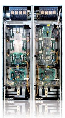
The SAMI STAR inverter units before the retrofit (above) and the new ABB industrial drive modules installed into the SAMI STAR cabinets (below).
