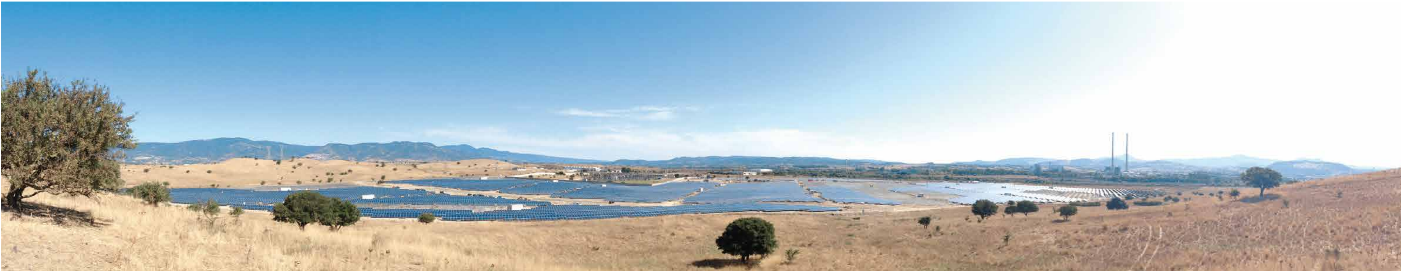
Ottana plant, Bolotana – Sardinia Region – Italy Total area: 404 500 m 2 or 45 ha; Total photovoltaic modules: 103 240; Power rating: 24 879.6 kWp; Expected annual production: 40 000 000 kWh; Reduction in CO 2 emitted into the atmosphere: 20 000 Tons; TEP reduction: 7480 Tons
