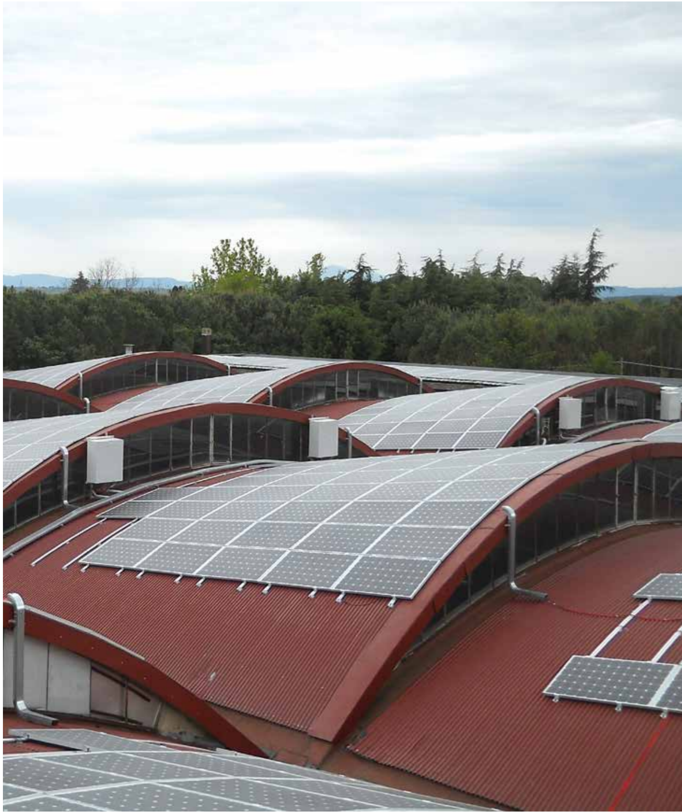
Castiglione Fiorentino plant, Arezzo – Tuscany – Italy Total area: 2350 m 2 ; Total photovoltaic modules: 1408; Power rating: 352.00 kWp; Expected annual production: 441 927 kWh; Reduction in CO 2 emitted into the atmosphere: 234.22 Tons; TEP reduction: 82.64 Tons
