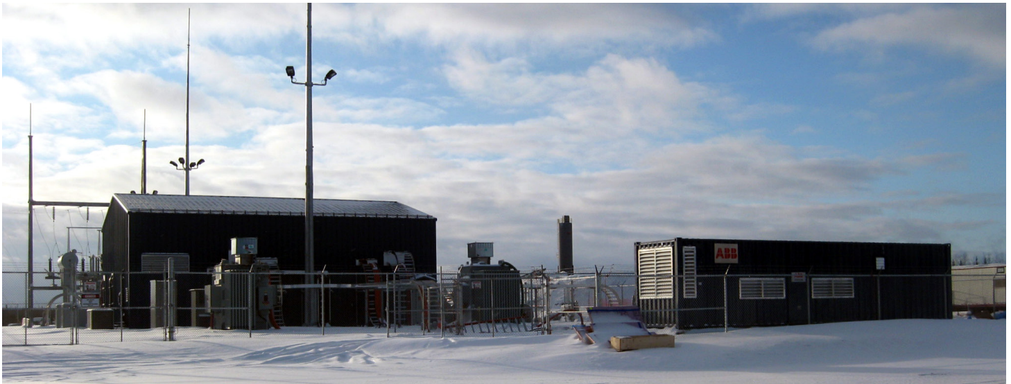
ABB's containerized STATCOM solution, with integrated transformer, installed in Ontario, Canada.
