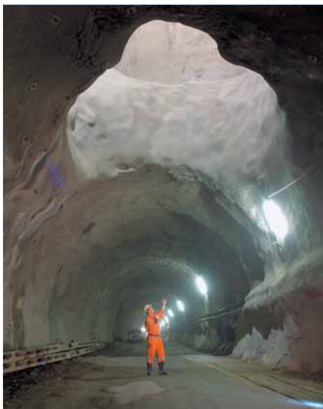
Ventilation tunnel at Sedrun. © AlpTransit Gotthard Ltd
