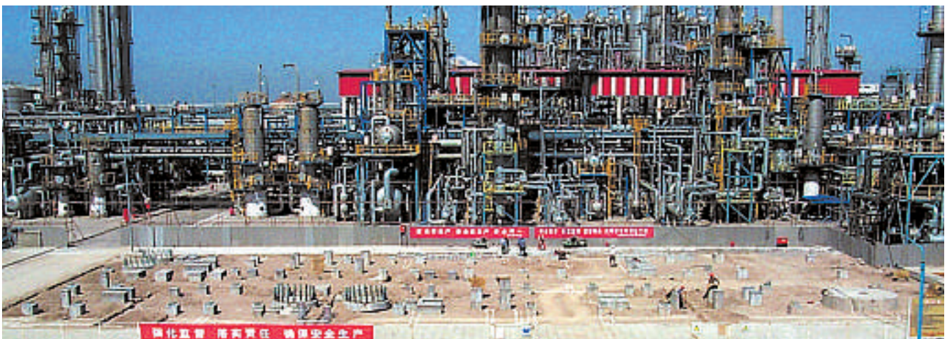
Construction site for the semi-commercial demonstration plants for CDHydro technology for front-end ethylene and Automet processes. Tianjin Petrochemical Complex, Tianjin, China.
