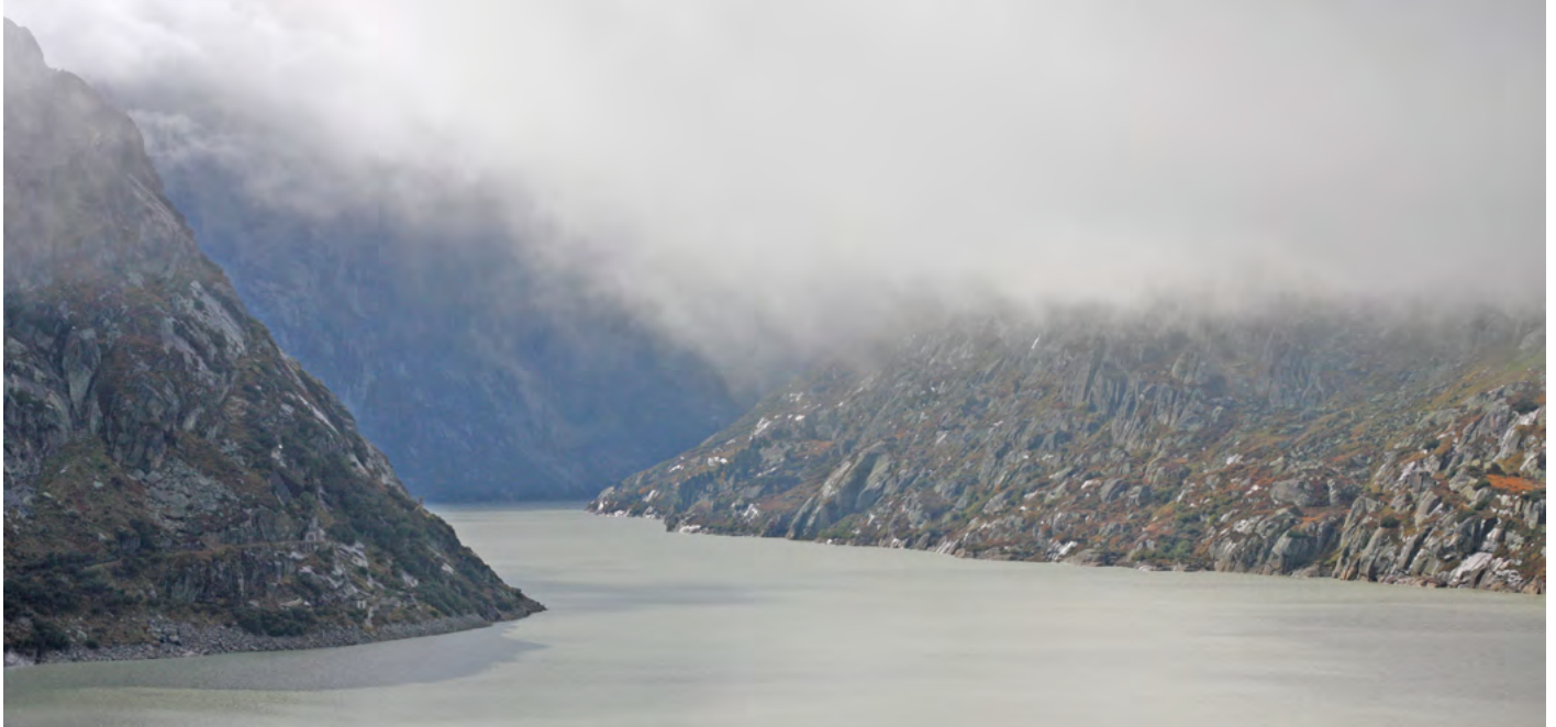
Upper lake of the pumped storage power plant Grimsel 2 in Switzerland
