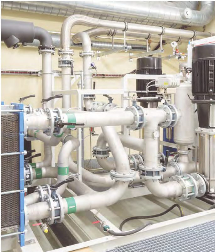
PCS 8000 cooling system
