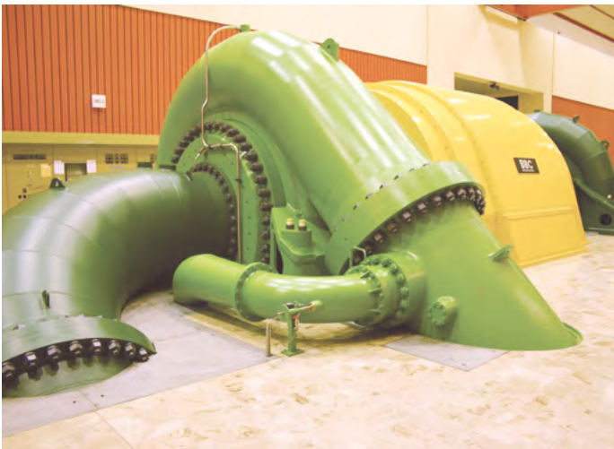
One 90 MW machine group comprising generator/motor, Francis turbine, and pump.
