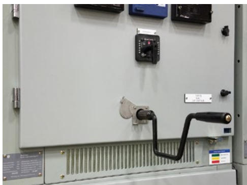
Figure 29. Racking Handle
