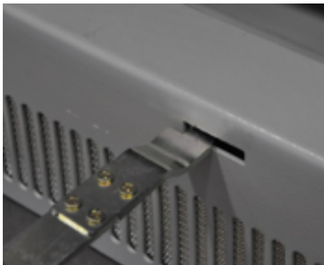
Figure 18. Operation Handle Fully Engaged into Switchgear Compartment
