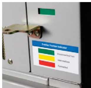
Figure 32. Disconnected/Test Position (Green)
