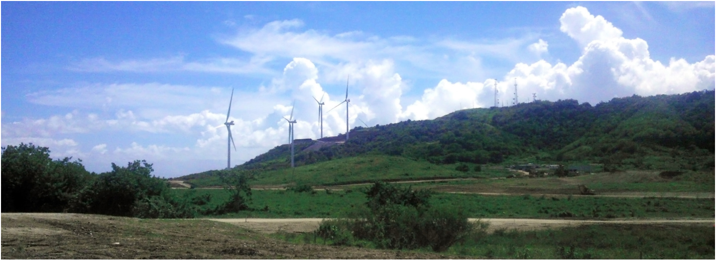
Punta Lima wind farm in Naguabo, on the windy eastern coast of Puerto Rico. The site provides 23.4 MW of renewable power generation to thousands of residents and businesses in the region.
